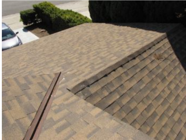
Roof is in overall good condition
