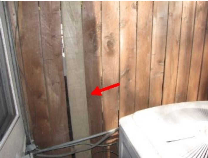
Loose fence board on right side of house
